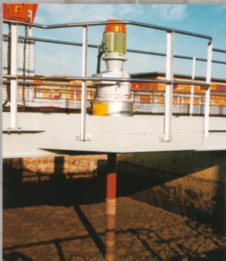
Anaerobic mixer
